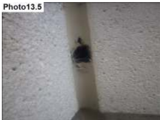
Sealant Failure Repair.
