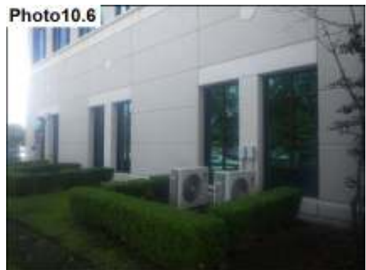
Back wall Lower Left Windows
