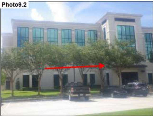
Back (North) Elevation Arrow marks area of leak.
