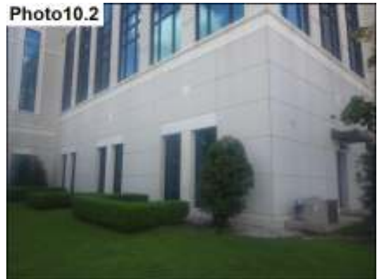
Back wall Lower Right Side Windows
