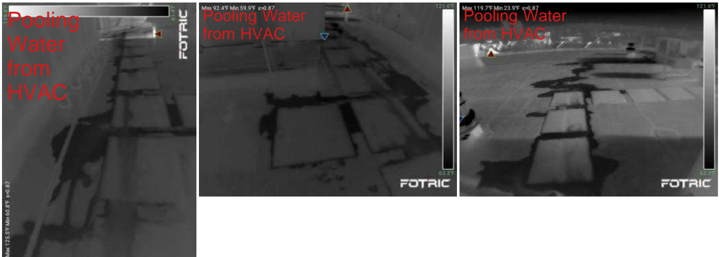
Photo #7: Infrared and Visual Photos of Roof Scan
