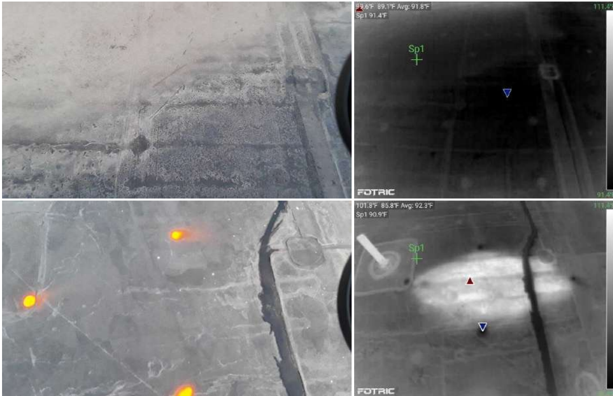
Photo #8: Infrared and Visual Photos of Roof Scan
