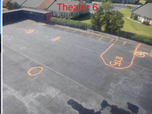
Photo #3: Roof Photos with Markings at Leak Locations
