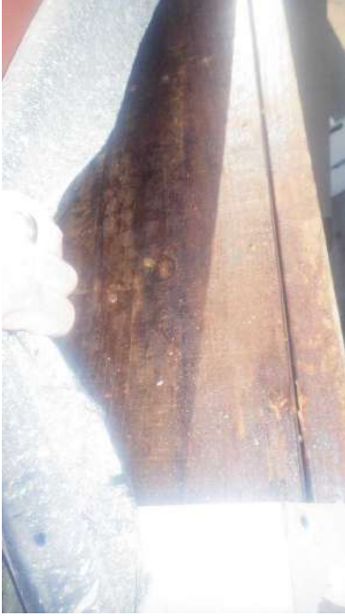
Photo #4: Damaged Gutter and exposed Roof System.
