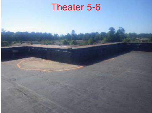
Photo #3: Roof Photos with Markings at Leak Locations
